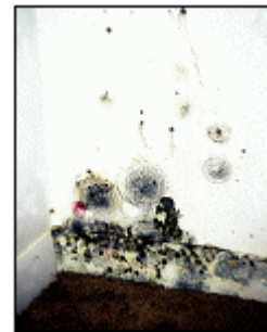
Mold damage on carpeting, baseboard and wallboard.
