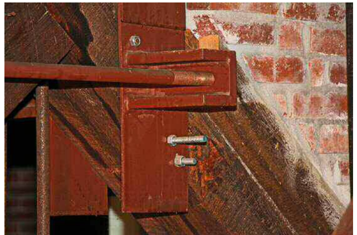
Attic Construction #4 Showing Turnbuckle Fixture Photo ID # 6861 Photo by Walt Roy
