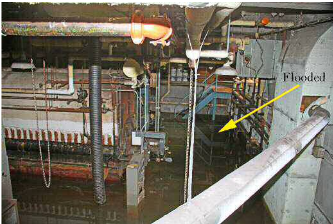
Science Building Boiler Room Note flooded floor Photo ID # 7322 Photo by Walt Roy
